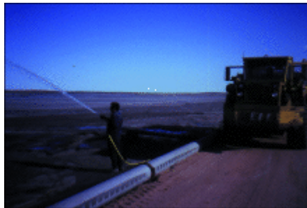
Photo: Pasminco Broken Hill Mine Pty Ltd Applying chemical sealant to stabilise the surface of tailings.
